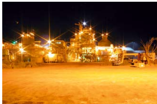
22 Sunrise Dam beneficiation plant (Anglo Gold Ashanti)
