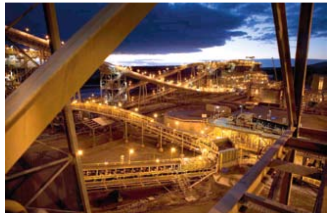
20 Boddington gold extraction plant (Newmont)
