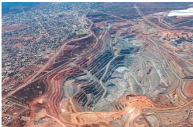
21 Boddington Mine beneficiation plant (Newmont)
